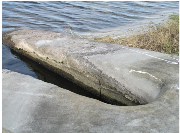
No Name Lake – Hairline cracks in concrete inlet structure
