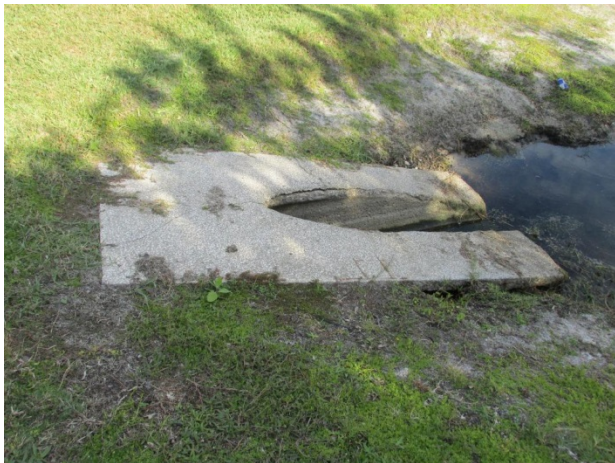
Gator Lake – Erosion at concrete inlet structure
