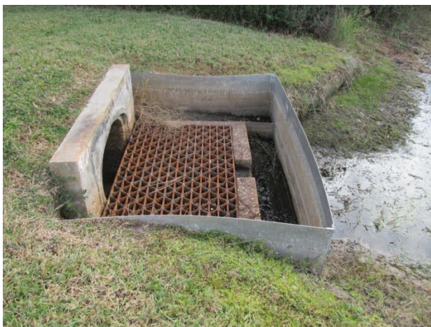
Deer Lake – Outlet structure
