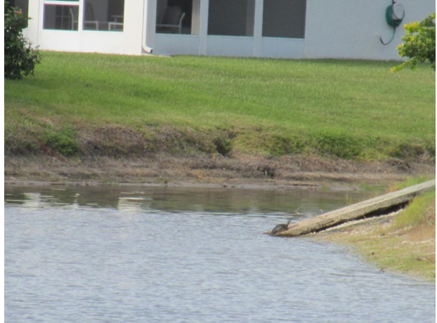
Crane Lake – Erosion evident
