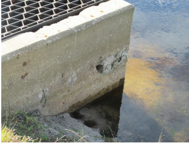
Quail Lake – Spalled concrete at outlet structure
