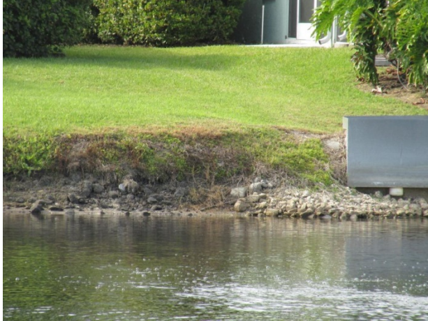
Crane Lake – Erosion evident
