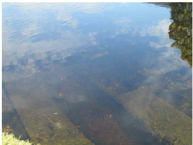
Heron Lake – Submerged concrete inlet structure
