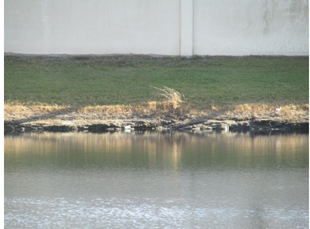
Egret Lake – Erosion evident
